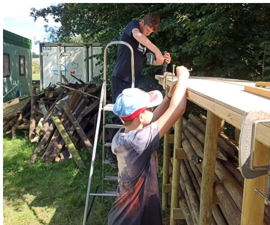
Building a pole shelter
