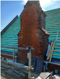
Roof repairs in action
