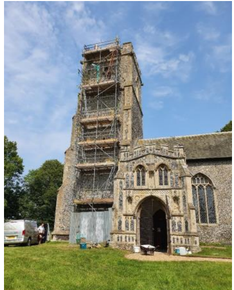
Oakley tower under restoration
