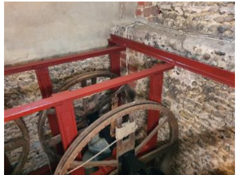
Oakley bell frame repainted
