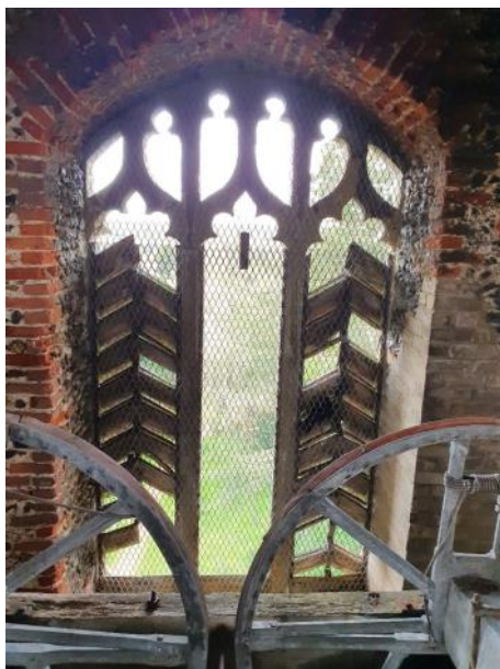
South louvres from inside the bell chamber
