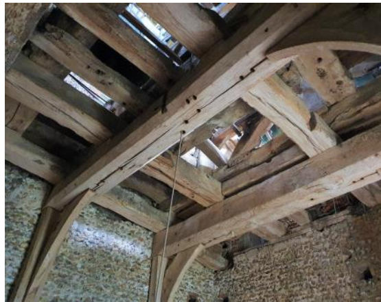
The bell frame which will be conserved, looking up from below.
