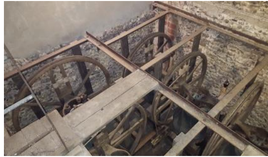
Oakley Bells hung in a 1958 steel frame
