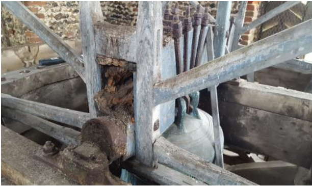
Rotten head stock on fourth
