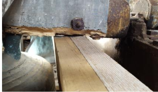
New Support under headstock of the treble bell
